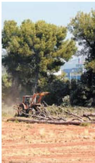
© Les obres a Can Bages. || J.G.
