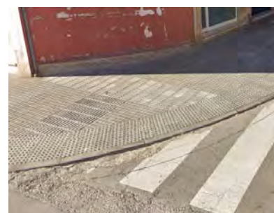
c. Puigvert (tram 77-ZED)
